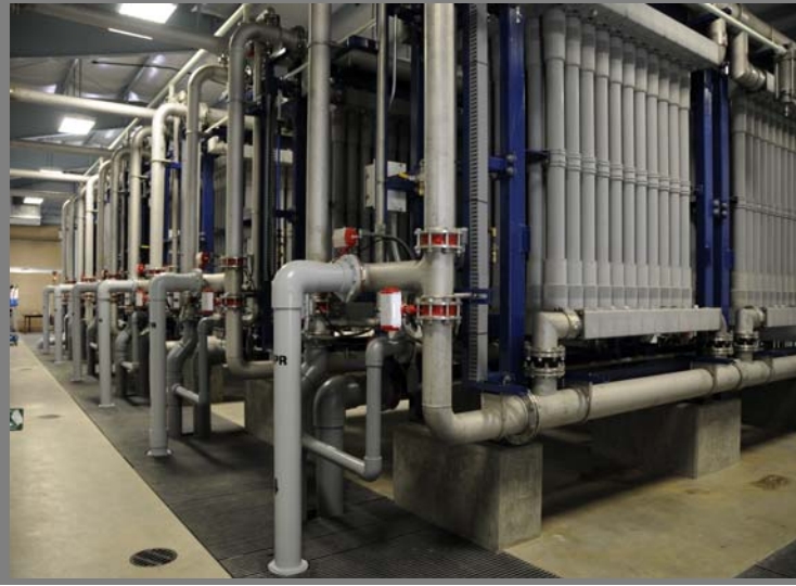
Completed installation of the 6 pressurized membranes inside the membrane building
